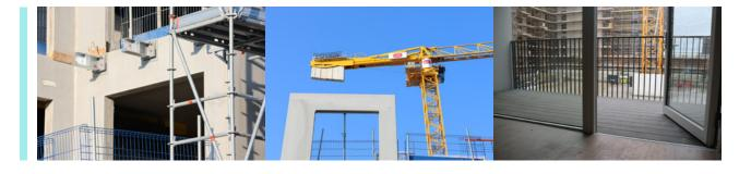
facilitated safer installations from within the building but also significantly reduced the balconies' embodied carbon by 34% compared to conventional concrete balconies, with approximately 20% of the thermal break surface area.
