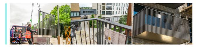
Our Remote Locker Device (RLD) was a key component in keeping balcony production and installation fast, efficient and minimally disruptive. The RLD is fixed onto a prefabricated balcony over preinstalled arms within the balcony Cassette®, the stubs already cast into the building's slab. The RLD then allows an installer to fix the arms to the stubs via a radio connection. Finally, after the balcony is secure, the remaining bolts can be safely fixed, and the Remote Locker can be removed.
